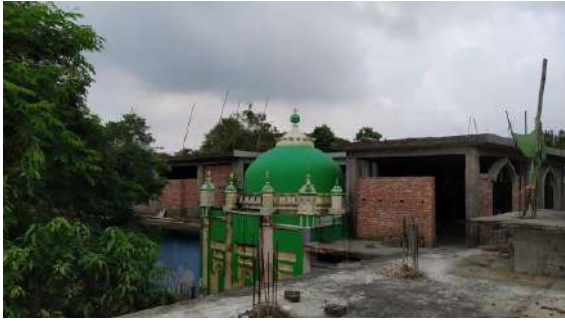
(Fig-13, present condition, source: authors)
