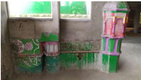
(Fig-11, present condition, source: authors)
